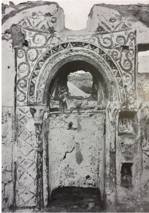
Apse niche in Room 1 (from MIFAO 59:2, Plate VI)
